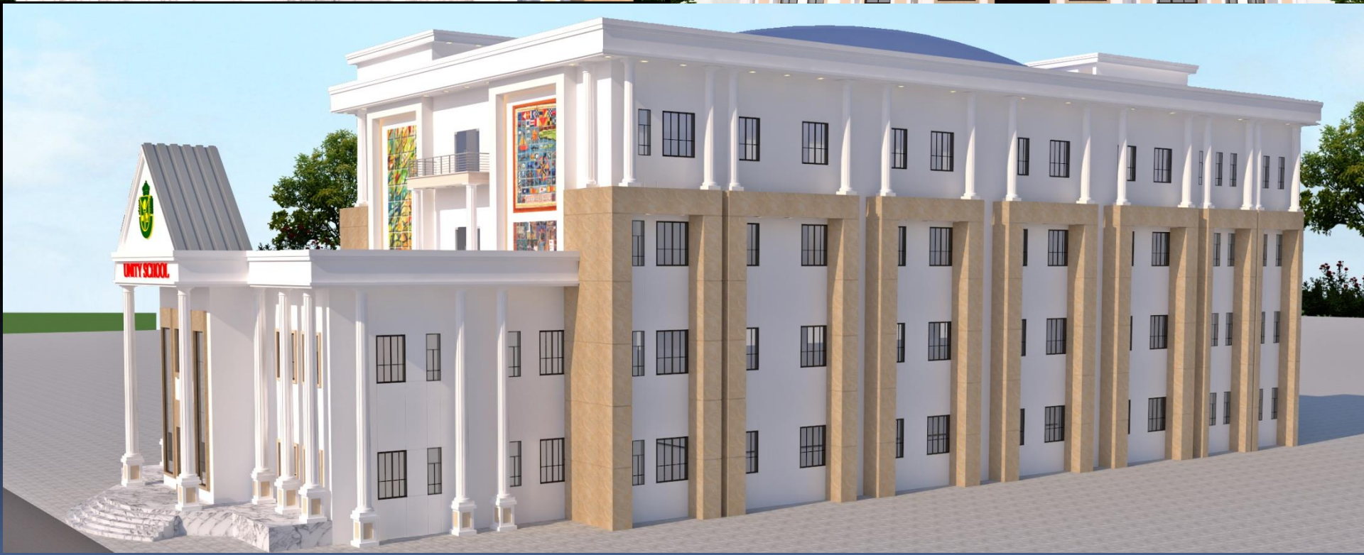
Unity School at Gonda (U.P.) - Construction going on
